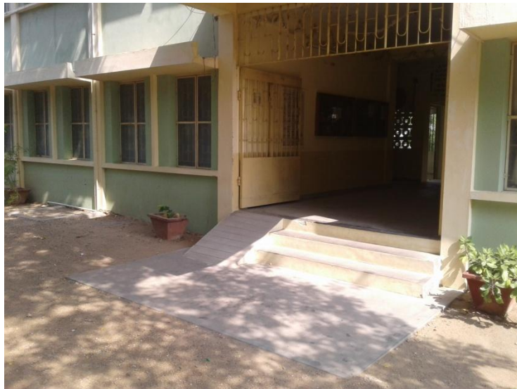
Ramps in College Campus
